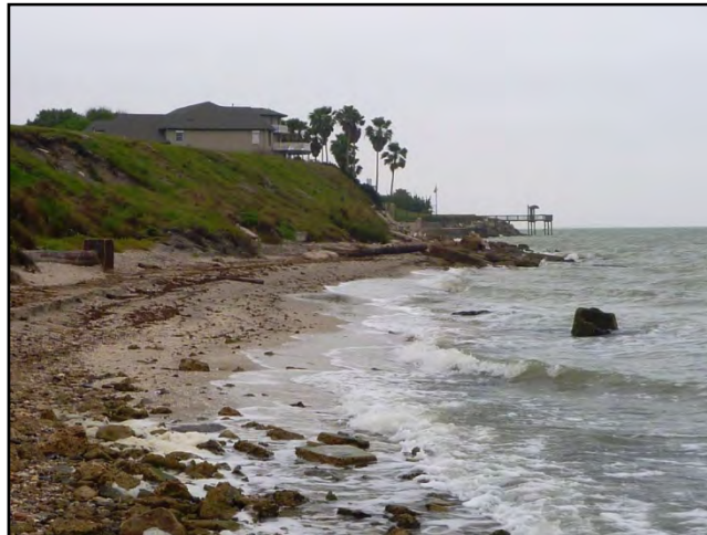
Fig. 2.19. Views of Ropes Park with A) sandy part of shoreline, B) access steps with signage, and C) storm water outfall and concrete rubble portion of beach in foreground and background with concrete debris in water clearly visible.
