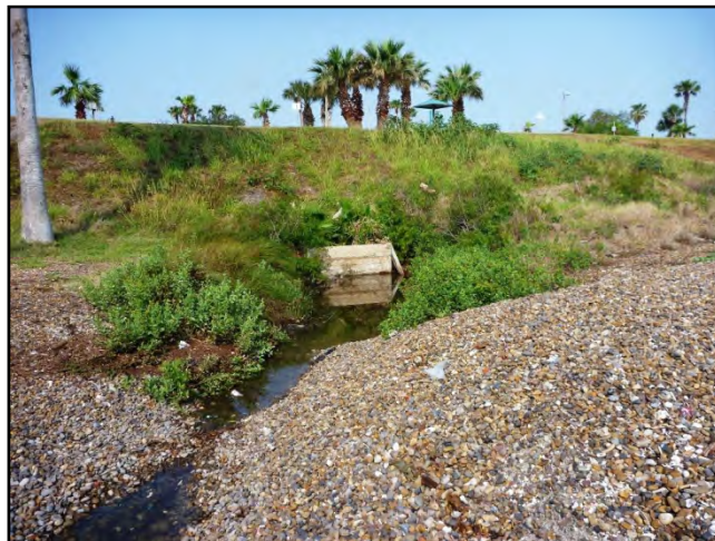
Fig. 2.17. Views of Cole Park at Oleander Point with A) rubble rock beach shoreline, B) access steps with signage, and C) one of the three storm water outfalls with stagnant water pools.
