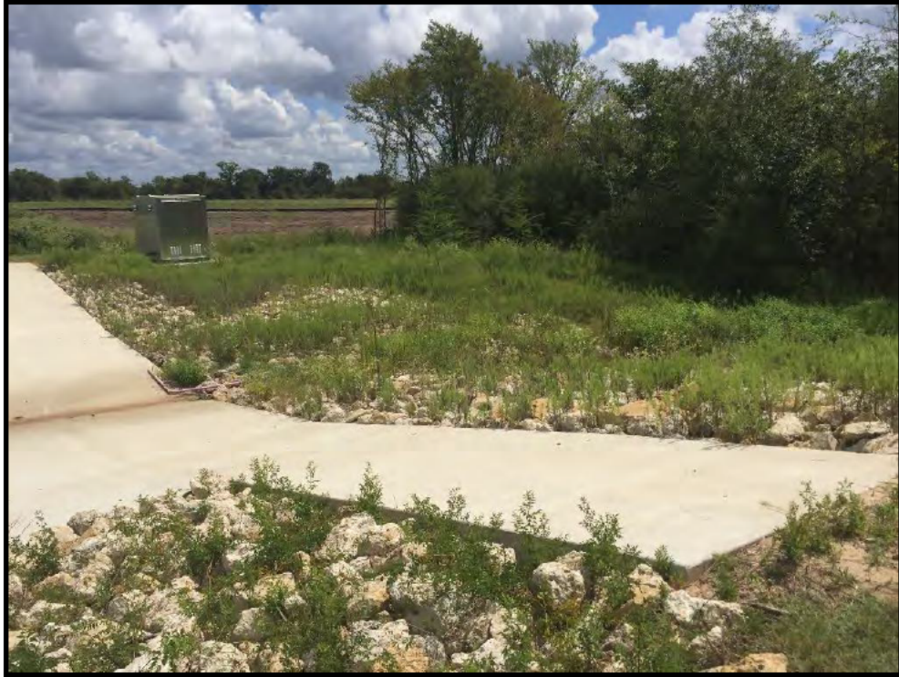
Photo 5: View east of reservoir spillway and un-named tributary to Lick Creek at the proposed Discharge/Diversion Point.
