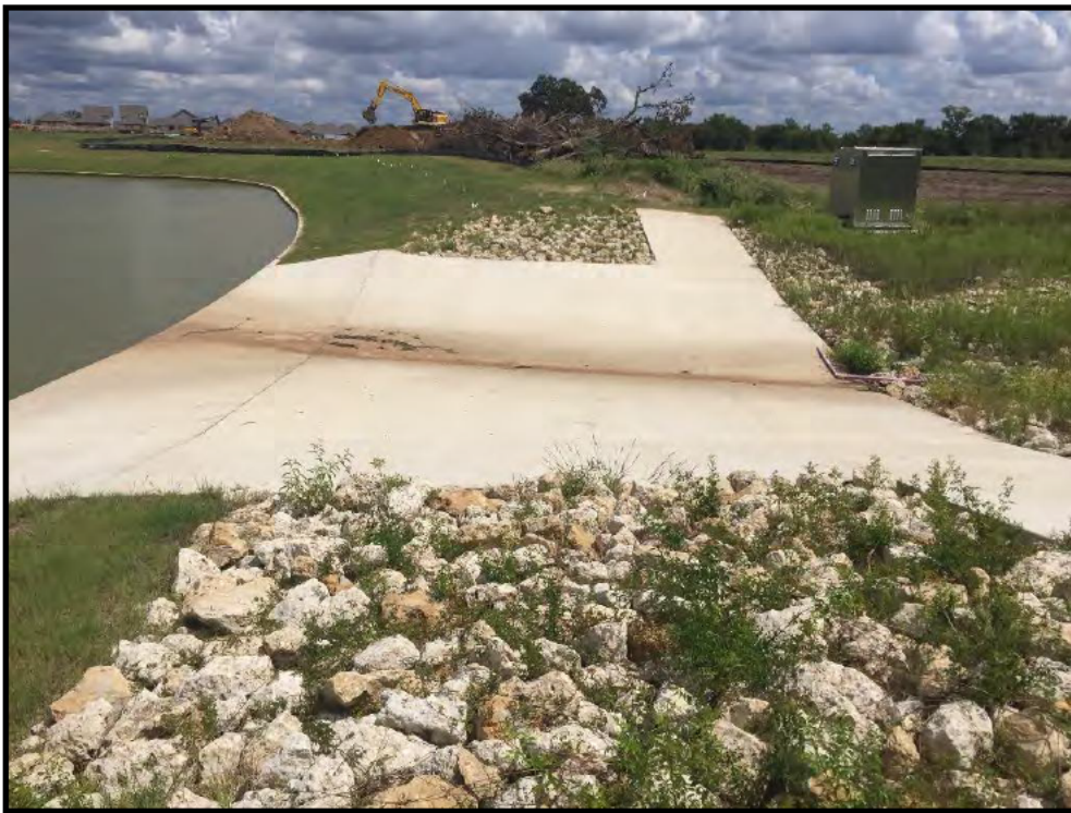
Photo 2: View northeast of reservoir spillway at the proposed Discharge/Diversion Point.
