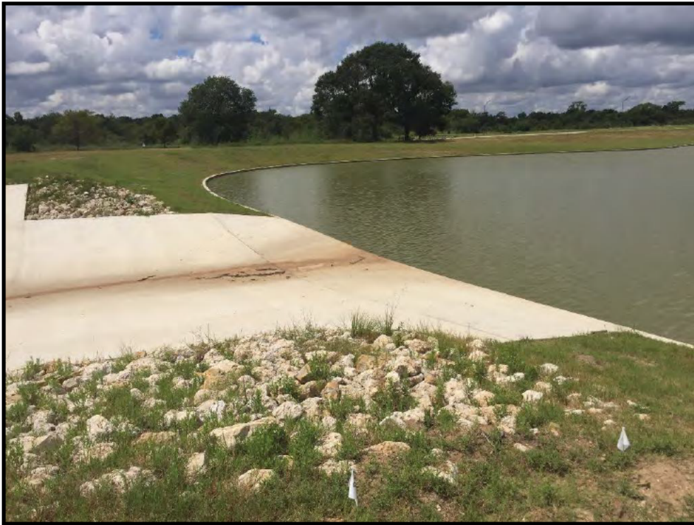
Photo 4: View west of reservoir spillway at the proposed Discharge/Diversion Point.
