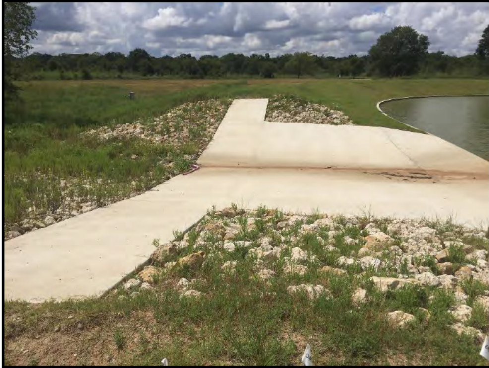
Photo 3: View southwest of reservoir spillway at the proposed Discharge/Diversion Point.
