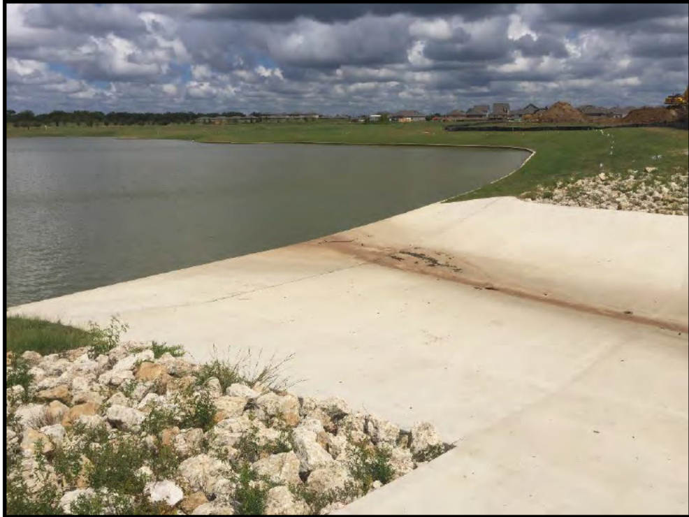
Photo 1: View north of reservoir spillway at the proposed Discharge/Diversion Point.
