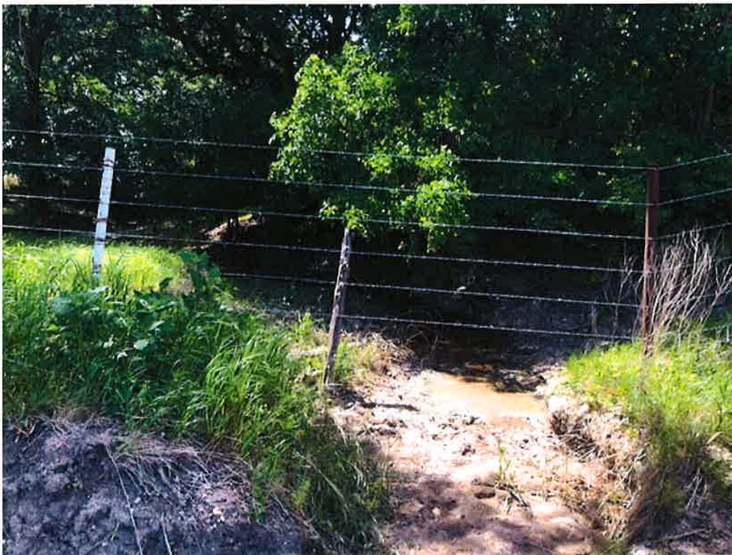
Photo 24: (Reach E-E') Downstream Limit E' Looking Downstream
