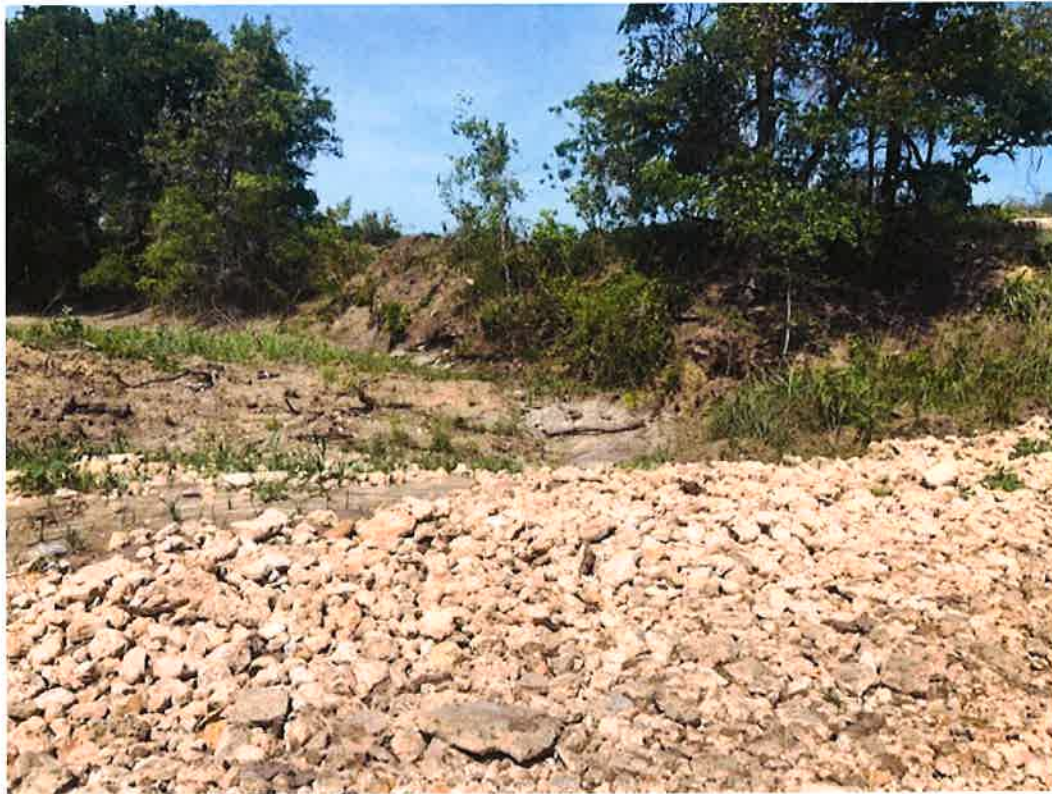
Photo 10: (Reach B-B') Upstream Limit B Looking Downstream
