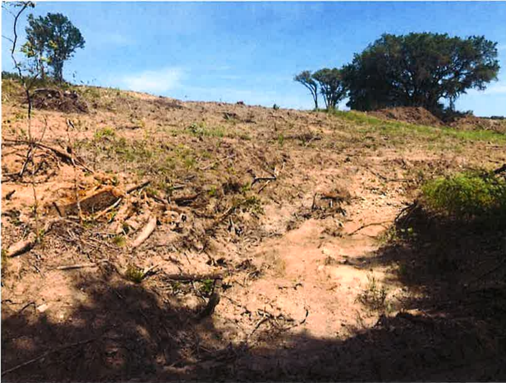
Photo 23: (Reach E-E') Downstream Limit E' Looking Upstream
