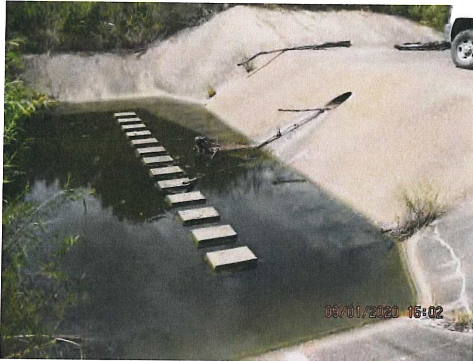
All-99R (3) top drop toward inlet of pond
