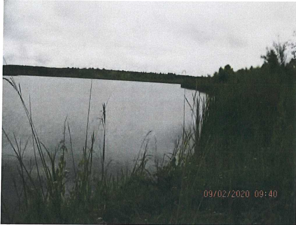
CIII-74R inlet (1) inlet looking east
