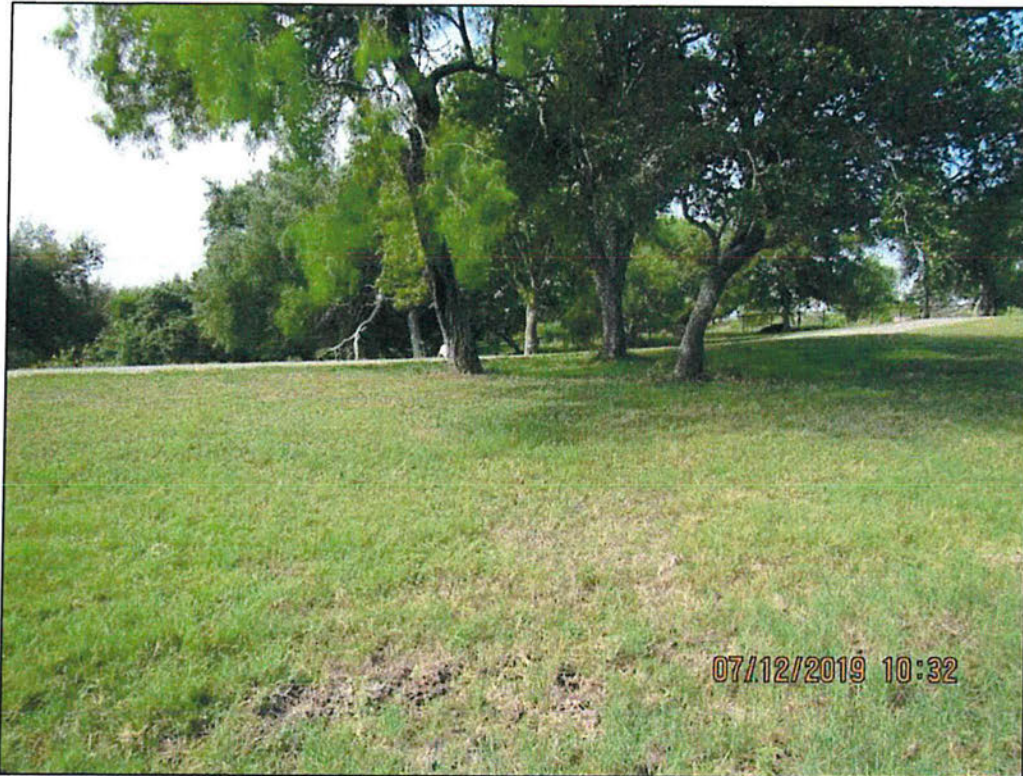
Photo 29 – Emergency spillway approach. Looking downstream. Note large trees in spillway flowpath.
