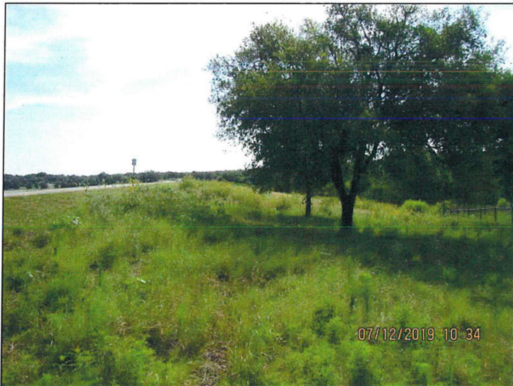
Photo 10 – Downstream slope. At right end of dam. Looking left.
