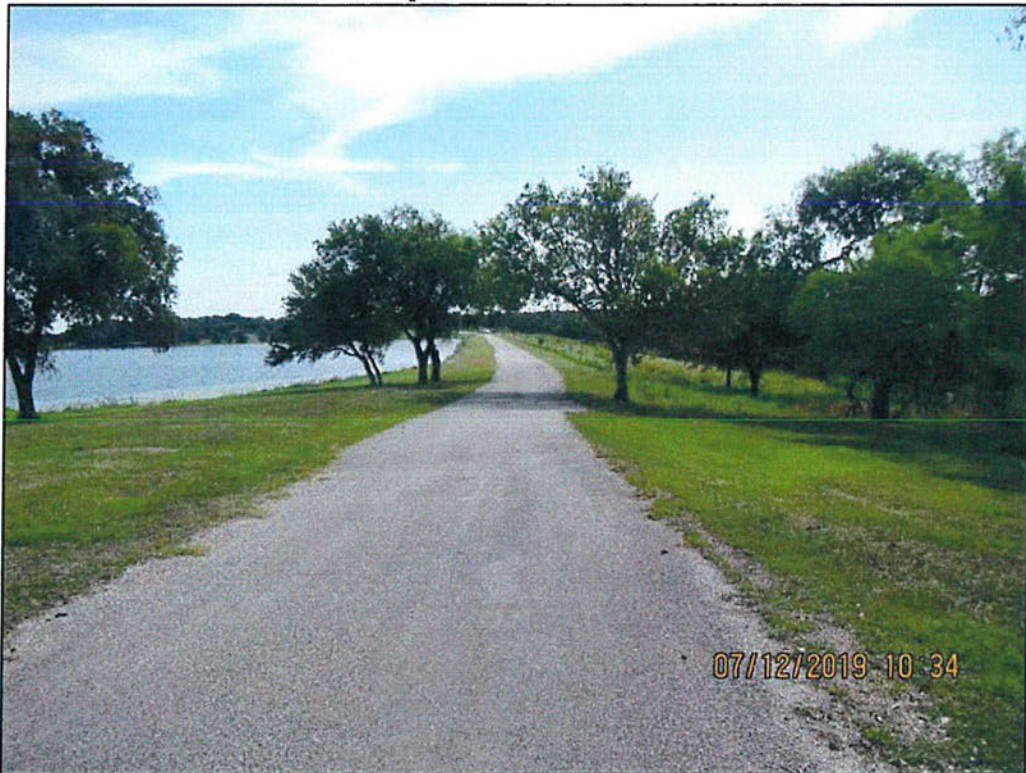
Photo 2 – Crest. At right end of emergency spillway. Looking left.
