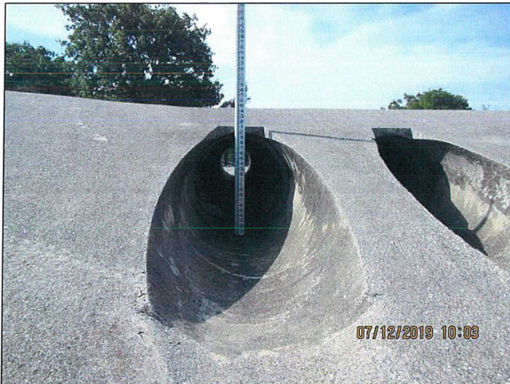
Photo 20 – Service spillway. Upstream culvert inlet. Eighteen 2-foot circular concrete culvert pipes.
