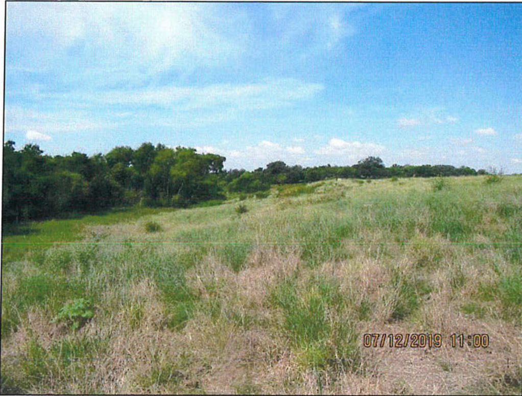
Photo 11 – Downstream slope. At service spillway. Looking right.
