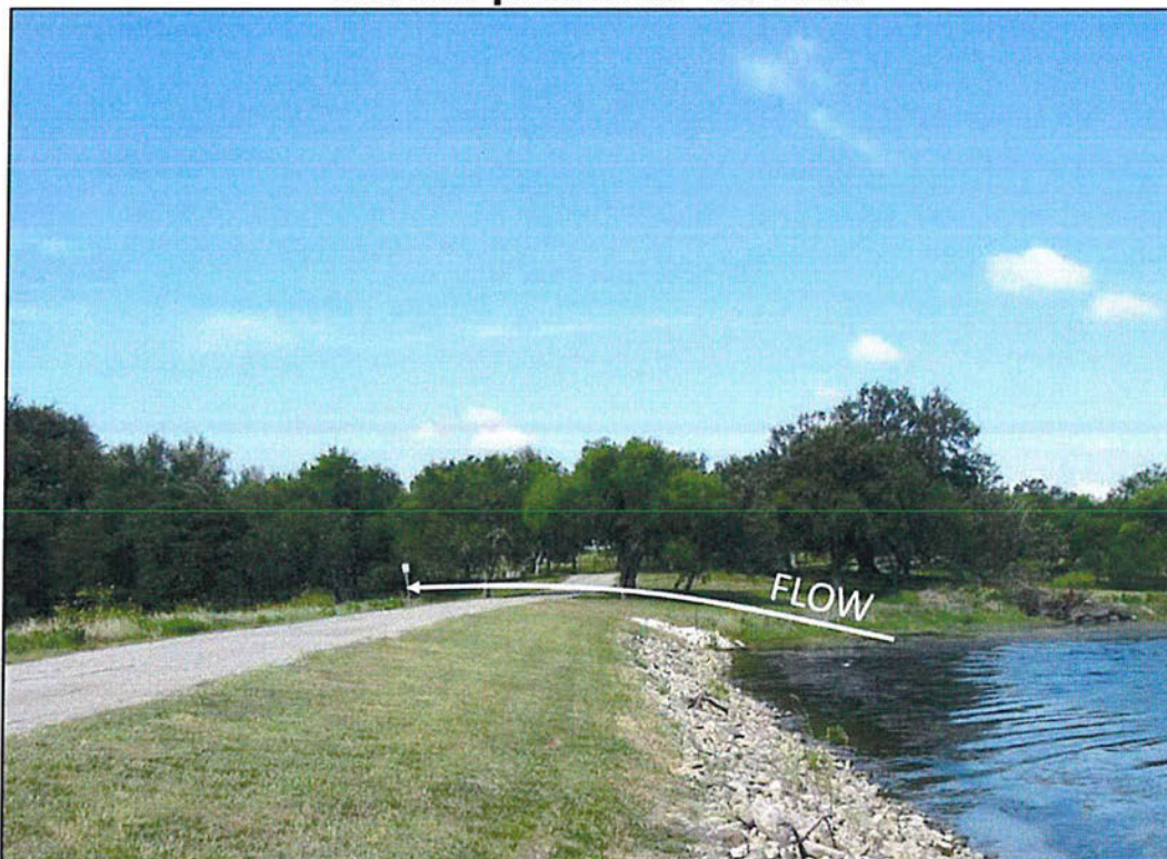
Photo 28 – Emergency spillway. At mid dam looking right.
