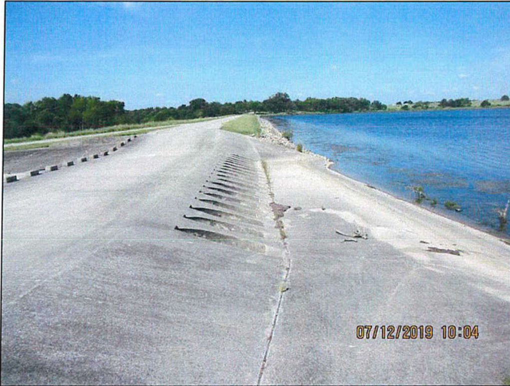
Photo 19 – Service spillway. At left end looking right.
