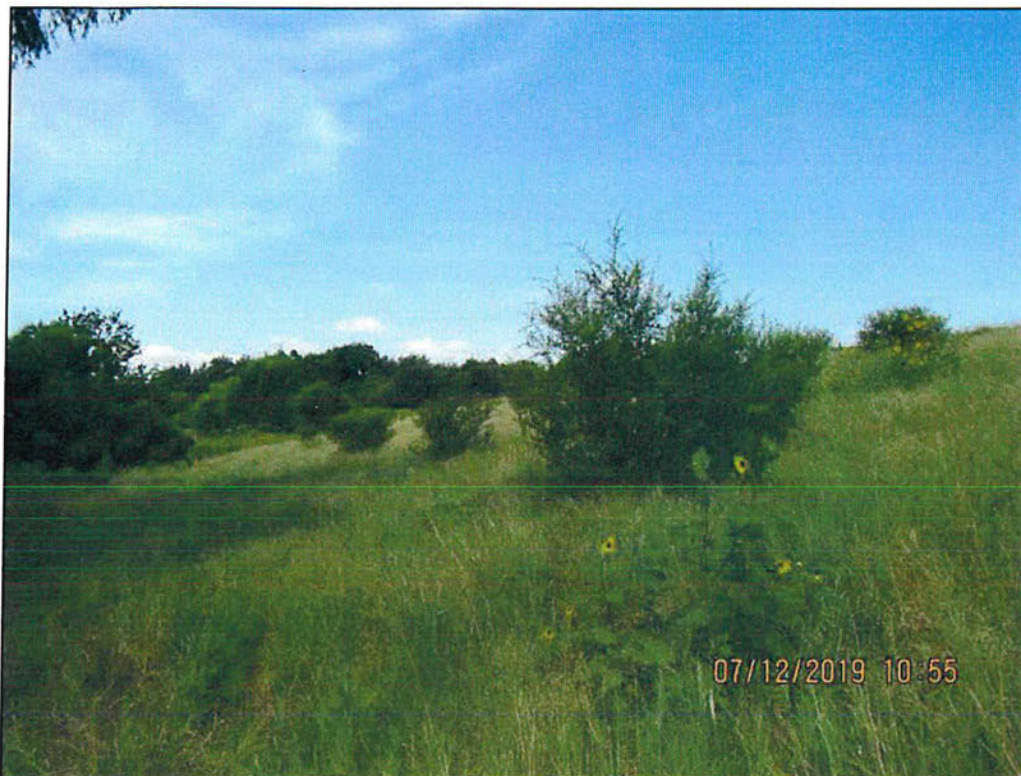
Photo 13 – Downstream slope. Mid embankment. Looking right. Note trees and brush.
