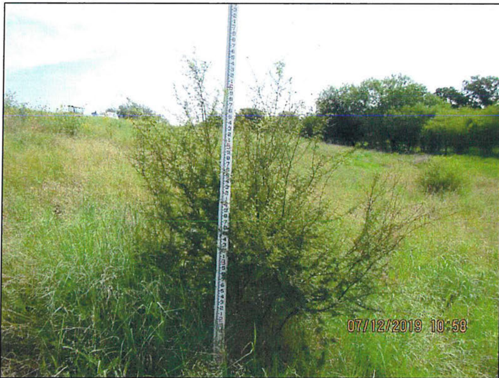
Photo 12 – Downstream slope. Mid embankment. Looking left. Note trees and brush.
