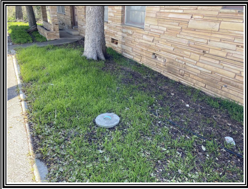
1. View of septic cover on the north side of the residential structure at the Sure Point Storage Tract on Highway 46 in New Braunfels, Texas.
