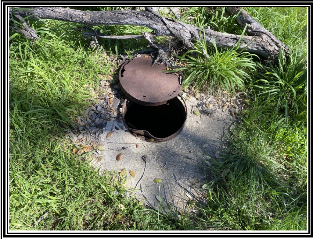
3. View of septic tank Feature S-3, located at 29-43-15; -98-10-37.5 in the west-central portion of the tract.
