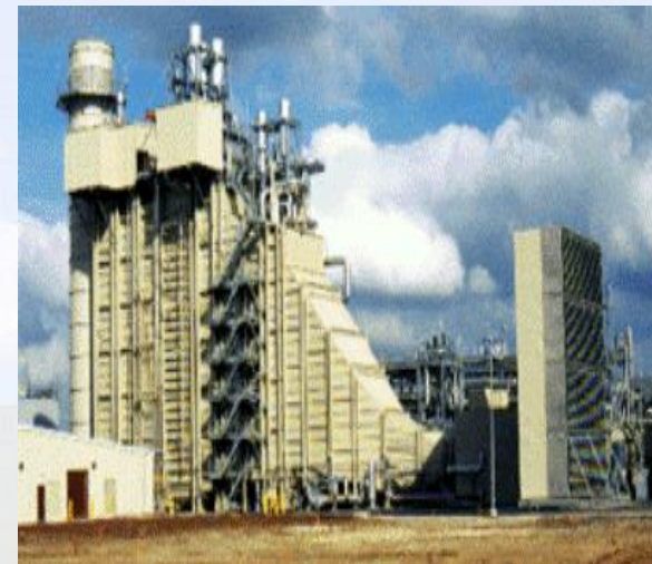
Power plant in Cleburne, Texas
